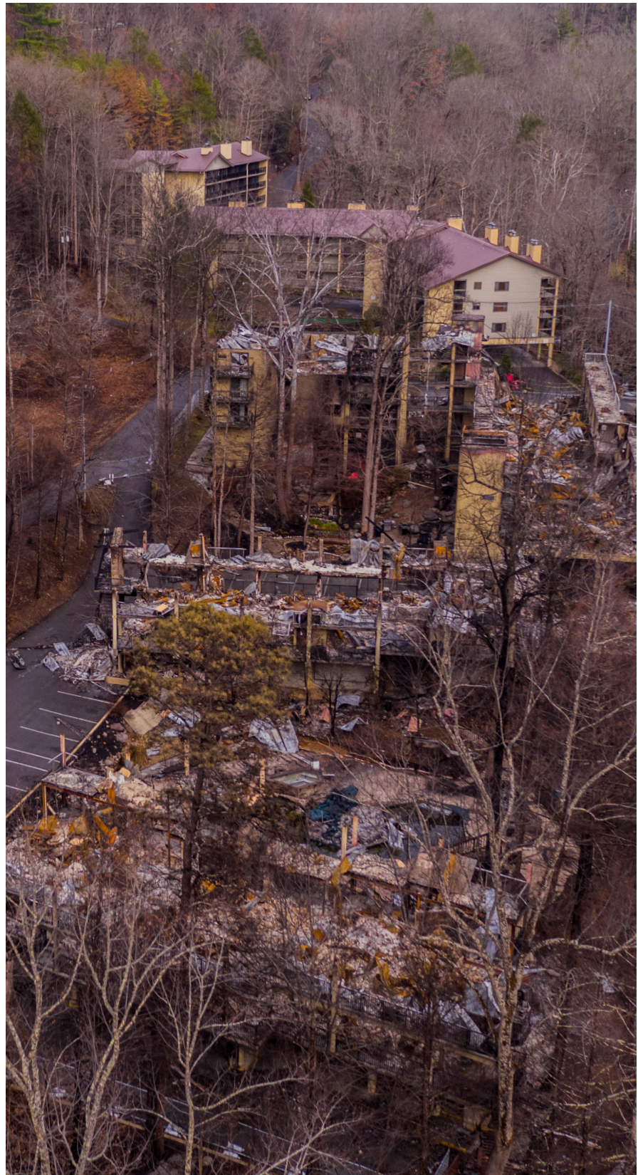
Gatlinburg fire damage.
