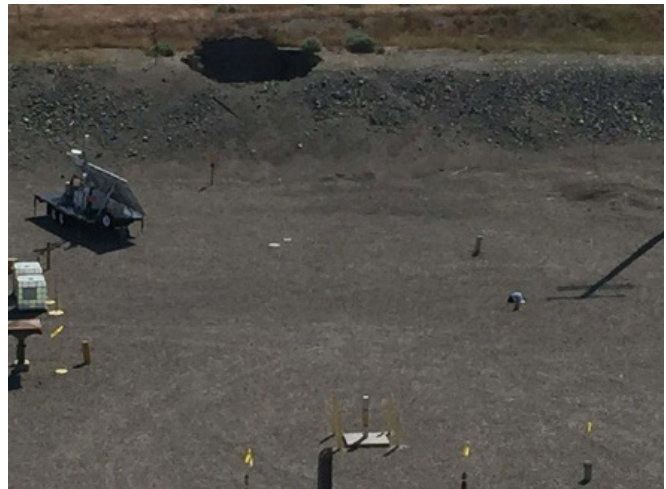
Collapse of PUREX Tunnel 1.
